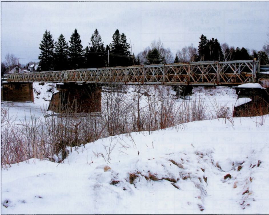
Figure 10. Goulais River's Bailey Bridge
